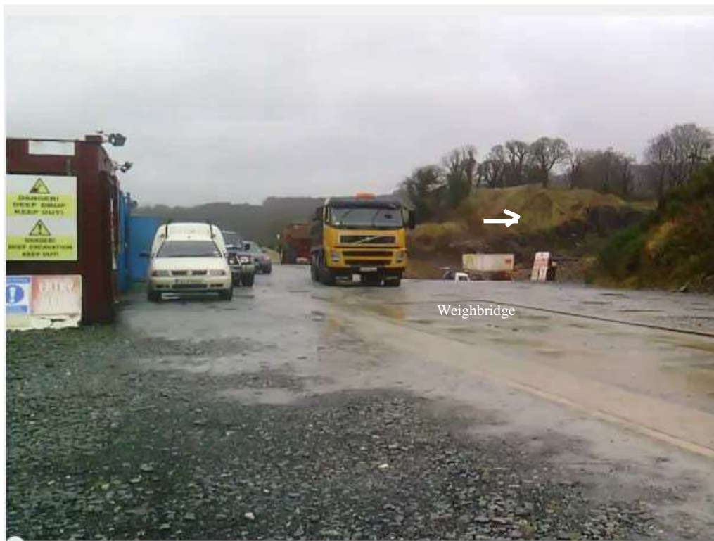
Plate 2.4 QMA, Site offices, warning notices and weighbridge, arrow shows direction of Quarry Working Area (QWA)
